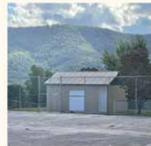
CHAIN LINK FENCE
